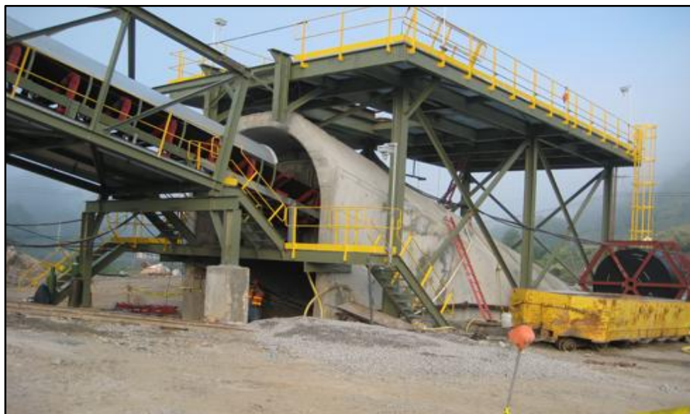
Figure 14: Example of a Slope Portal Transporting ROM Coal to Preparation Plant
