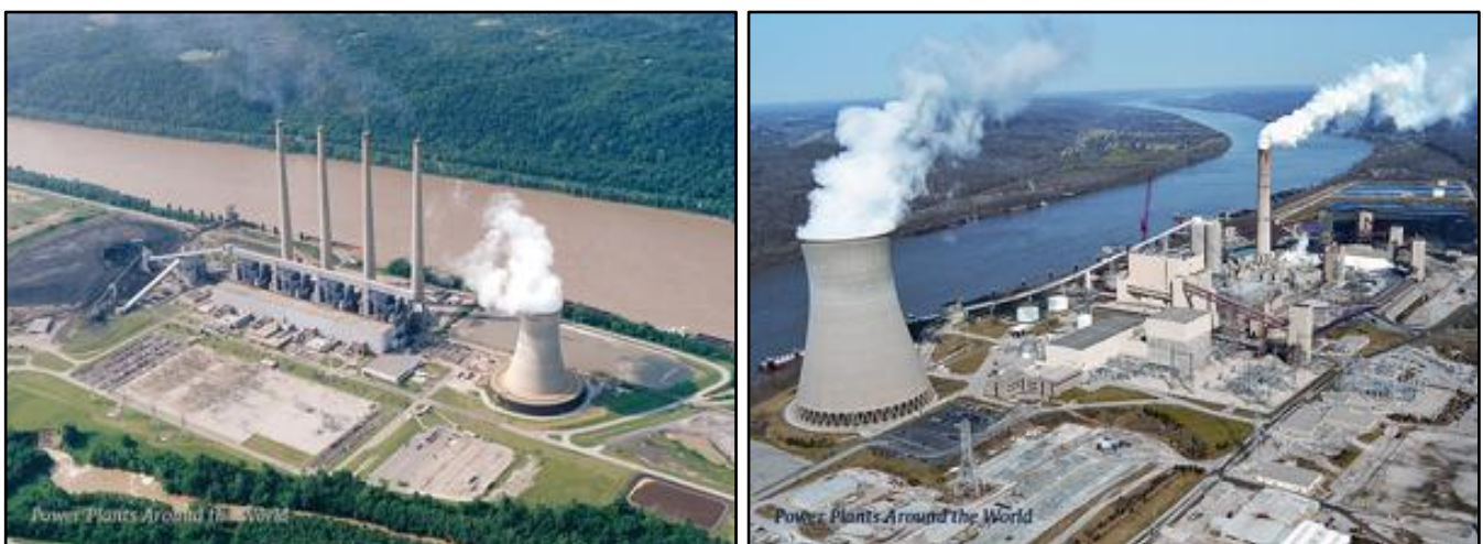
Figure 9: Typical Modern Coal Fired Power Plants on the Ohio River
