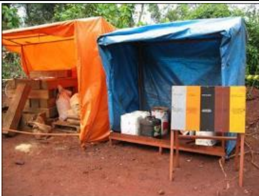
Large diameter coring operations – safe storage of drill consumables and recycling
