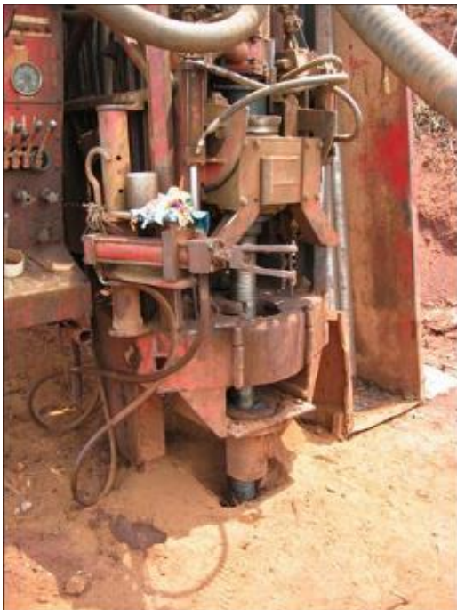
Infill RC operations – equipment is old but drilling penetration rates are high
